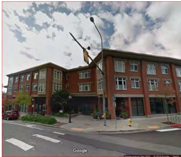
Intersection at 7th Avenue and Market Street
