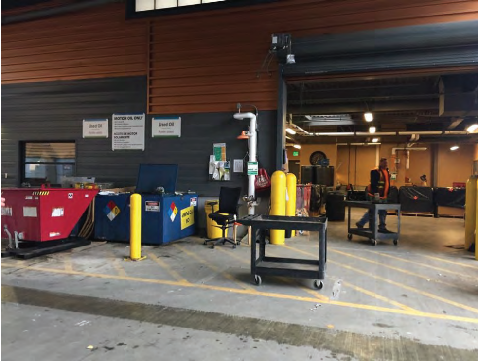
Figure 5 Hazardous waste drive thru drop-off station.
