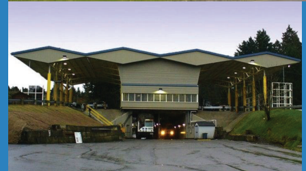
The Houghton Transfer Station in Kirkland
