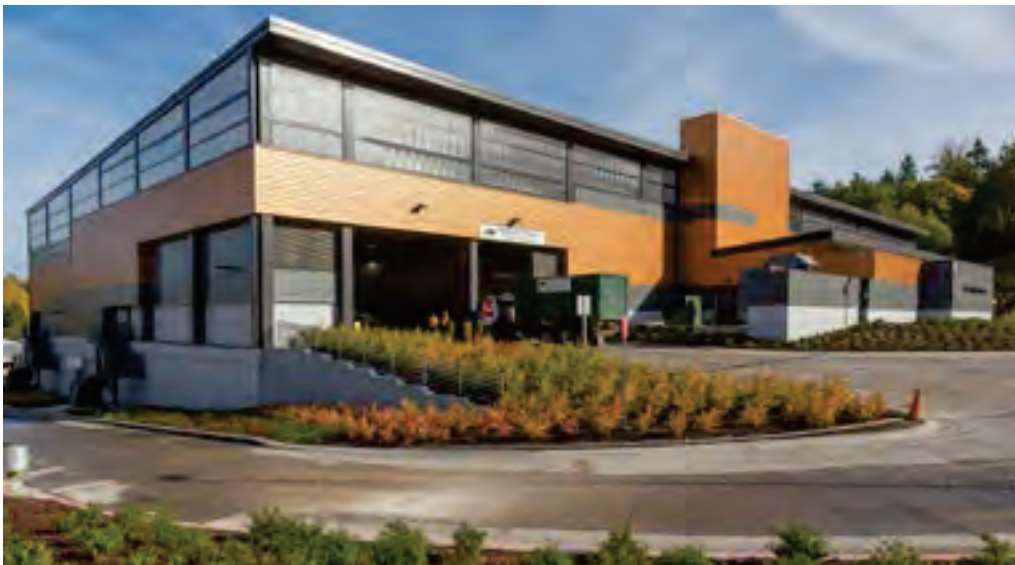
Factoria Recycling and Transfer Station
