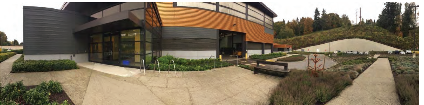
Figure 4 Panoramic view (distorted) of front door entrance portico extending to visitor parking and retainer wall.
