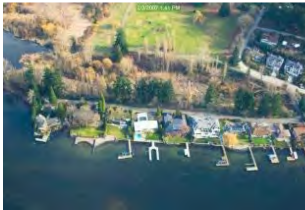
Piers near Juanita Bay
