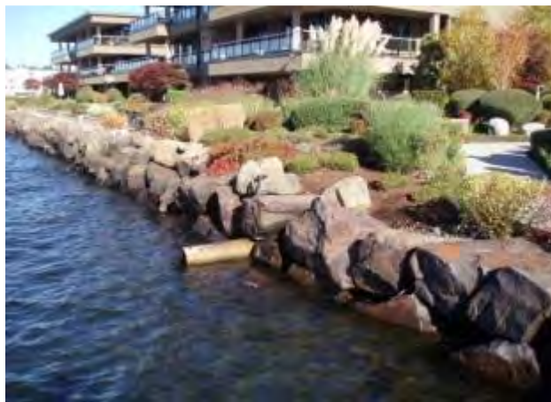
Bulkheads along the lake
