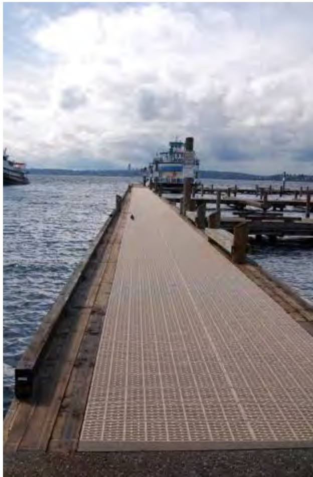
Marina Park pier with grating decking
