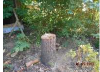
Illegal tree removal on an active development site
