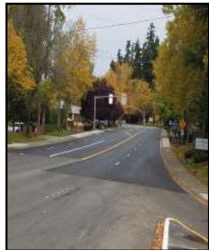
Pavement/lane striping complete
