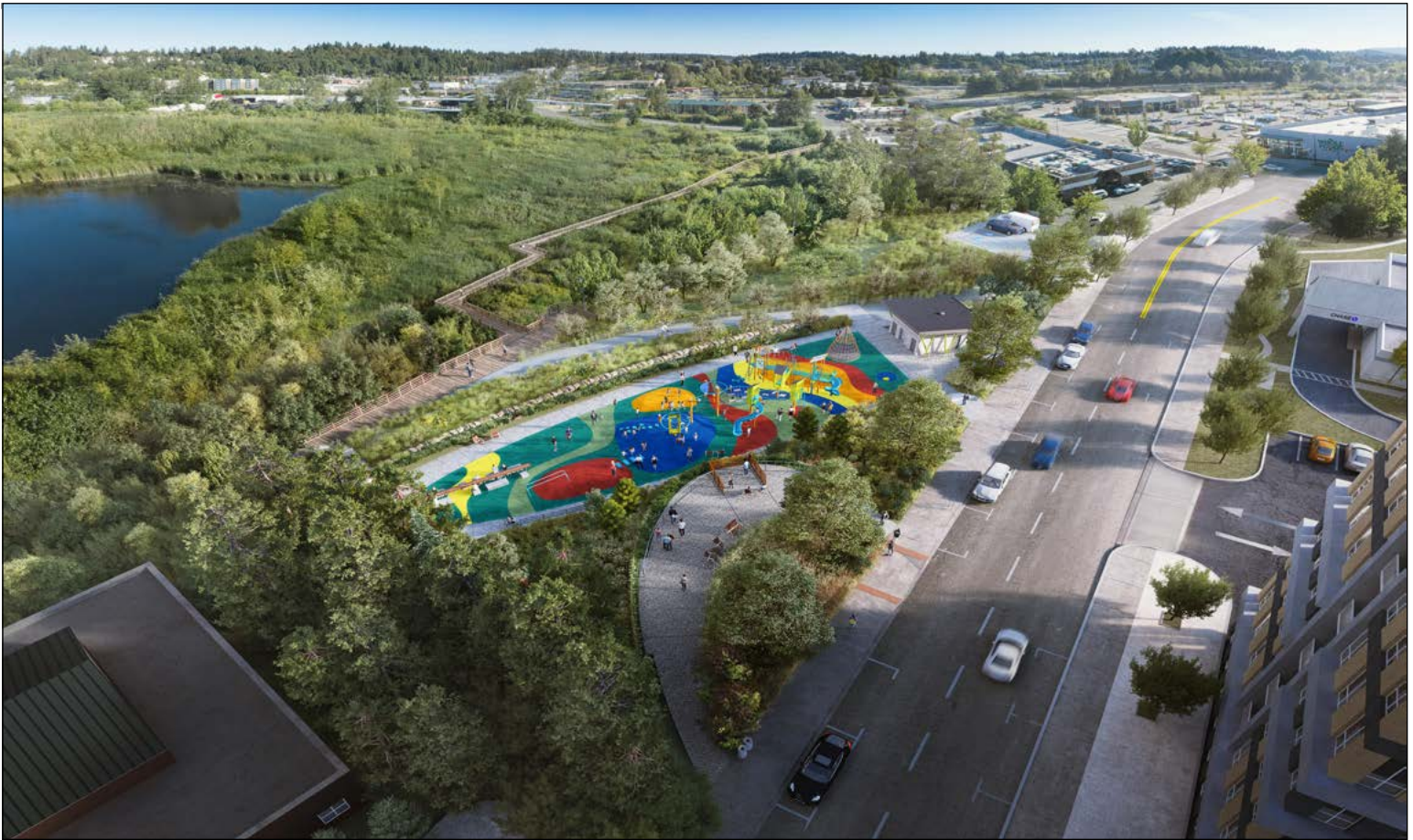
The transformation of Totem Lake Park into a regional destination began in April. Throughout the next year, contracted crews will build restrooms, picnic areas, boardwalks that connect to the Cross Kirkland Corridor and a playground that is accessible to all abilities.
