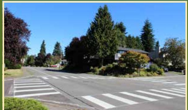
*Repainted crosswalk markings and replaced damaged curb for safe route to school along NE 84th Street from NE 139th Street to NE 141st Street*
