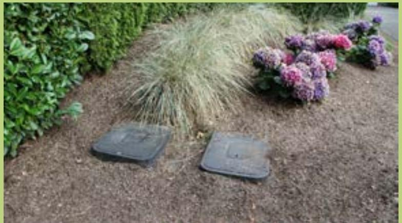
*A good rule of thumb is to keep 3 to 5 feet of cleared area around your water meter.*
